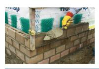
Follow good masonry practices, use clean water, erect a sample panel, evaluate mortar colors, use clean tools, be aware of weather conditions and choose the correct mortar type.
